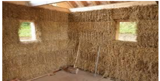
Image 5 – House insulated with Straw Bales
